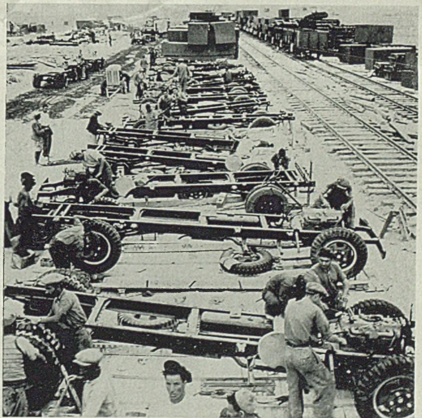
TRUCKS FOR RUSSIA: Military transports for the Red Army are assembled beside railroad tracks in the open desert in Iran while a special plant is constructed for the Army Ordnance Department. The plant is one of three, two in Iran and one in India, constructed by General Motors for assembling several makes of military vehicles, including Chevrolet and GMC trucks
