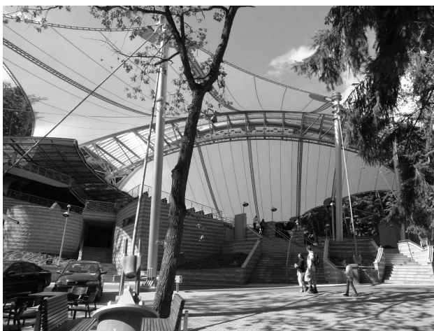
Fig. 15. The roofing of the Forest Opera in Sopot (author)
