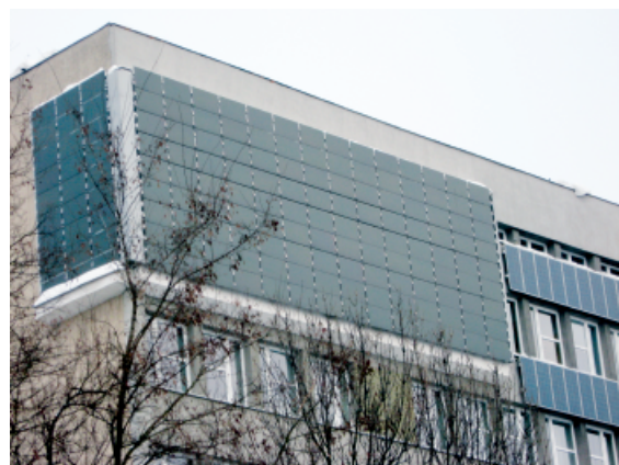
Figure 11. PV modules installed on facade – Environmental Engineering Faculty building in Warsaw (photo J. Tymkiewicz)
