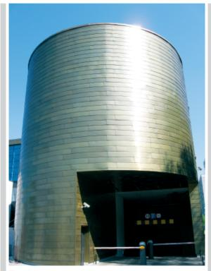
Figure 4. Fragment of the added part of the PWST building covered with copper plate, Wrocław (photo J. Tymkiewicz)
