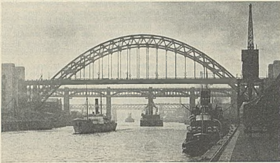
Abb. 5. Tyne-Brücken in Newcastle.
