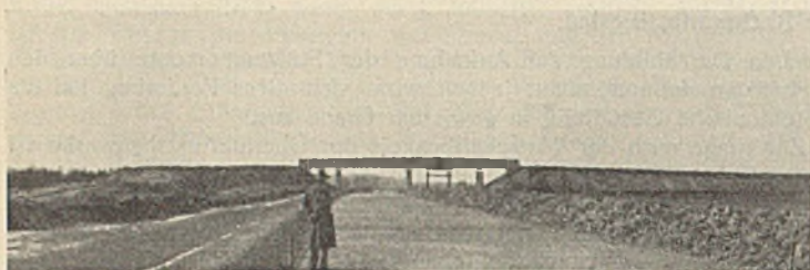
Abb. 5. Brücke 67 in km 67,4.
