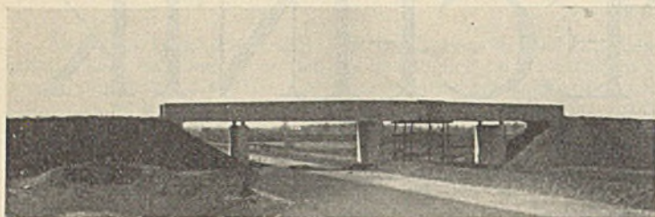
Abb. 4. Brücke 67 in km 67,4.
