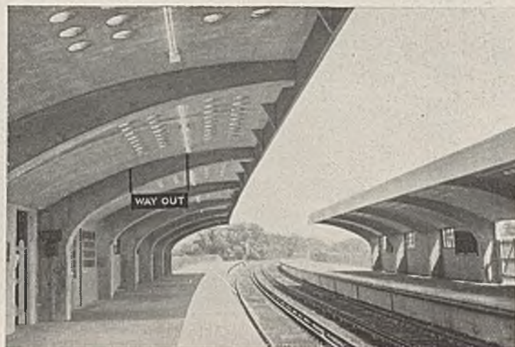
Abb. 31. Bahnsteigdach Malden Manor (Southern Railway), London.
