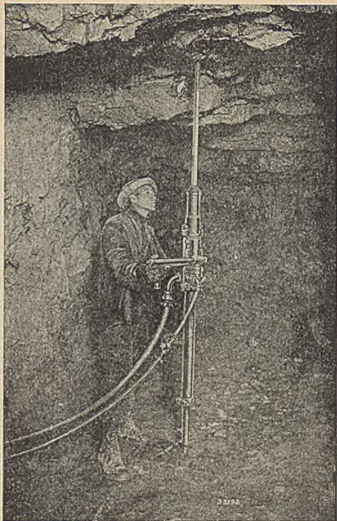
Fig. 8. —A stoper drill in operation. This type drill is widely used in underground mining work.
