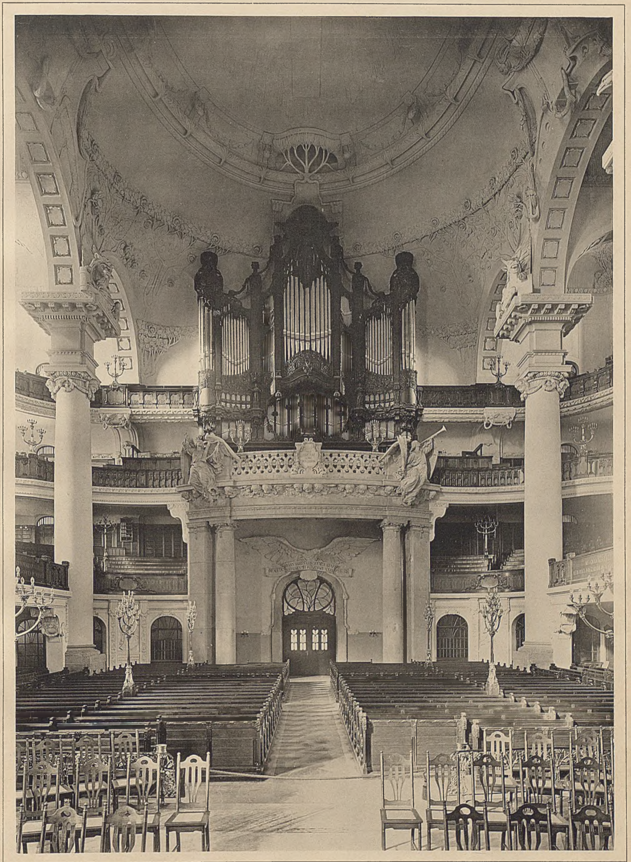
SCHILLING & GRÄBNER ARCH. 1898-1900
