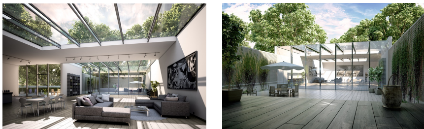
Figure 1.1: Pilot project. Hybrid timber-glass beams as load-bearing components of roof structure and conservatory (Authors: A. Kozłowska, A. Klich | AK 2 )
