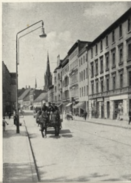
Betonstraße in Ratibor
