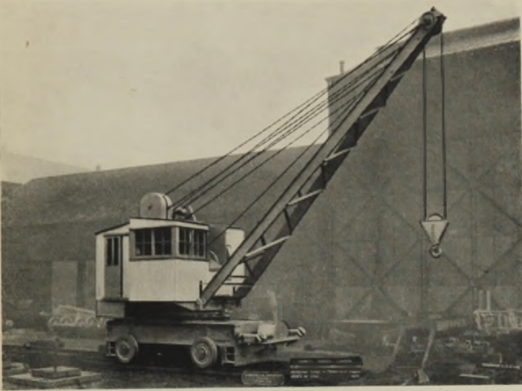
Ransomes & Rapier Ltd. 8-TON ELECTRIC LOCOMOTIVE CRANE.
