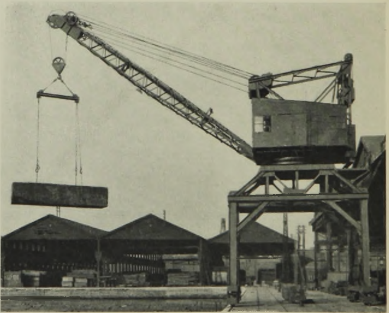
Sir William Arrol & Co. Ltd. 10-TON LEVEL-LUFFING CRANE LIFTING TIMBER.
