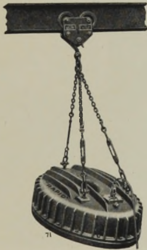
71 OVAL MAGNET SLUNG FROM TROLLEY.
