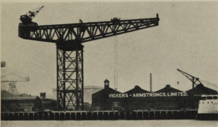
Sir William Arrol & Co. Ltd., Glasgow. 250-TON GIANT CRANE FOR FITTING OUT SHIPS.
