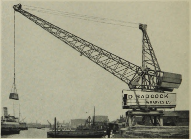
CRANK-OPERATED LEVEL-LUFFING CRANE.
