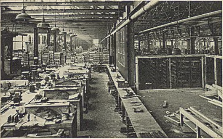
GENERAL VIEW OF 24-INCH CORE CONVEYOR.
