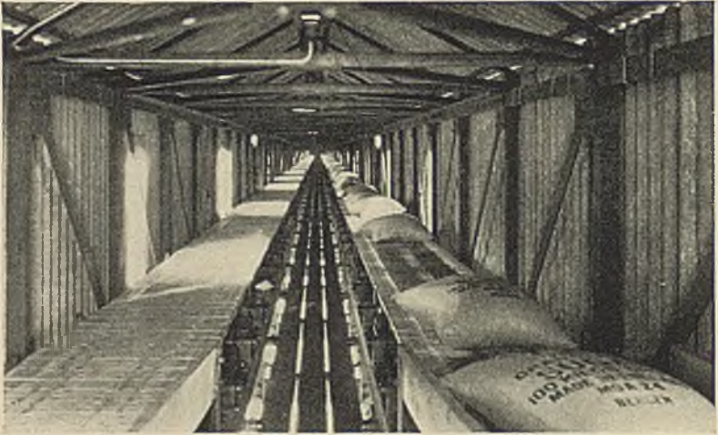
30-INCH TWIN SLAT CONVEYORS FOR SUGAR.
