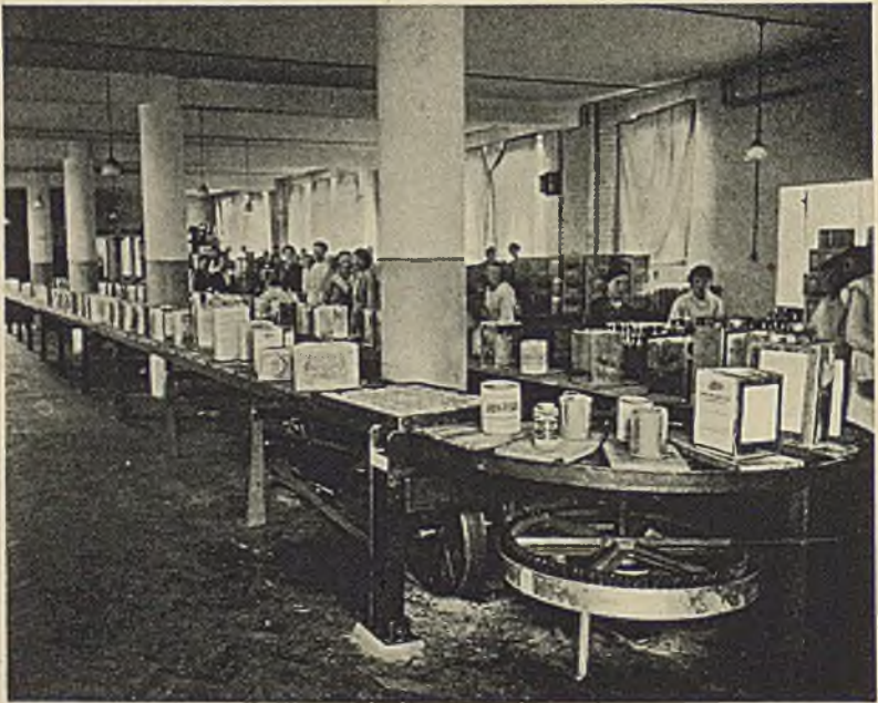
DOUBLE-SERVICE CONVEYOR IN FLOOR-POLISH FACTORY.
