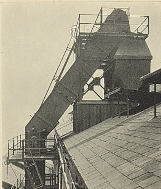
CRANKED COAL ELEVATOR.
