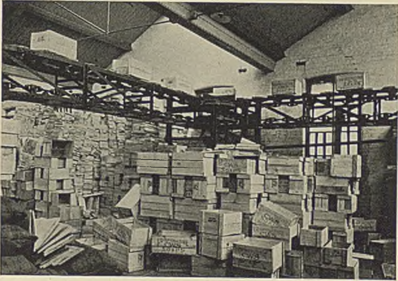
HORIZONTAL TURN IN SOAP-BOX CONVEYOR.
