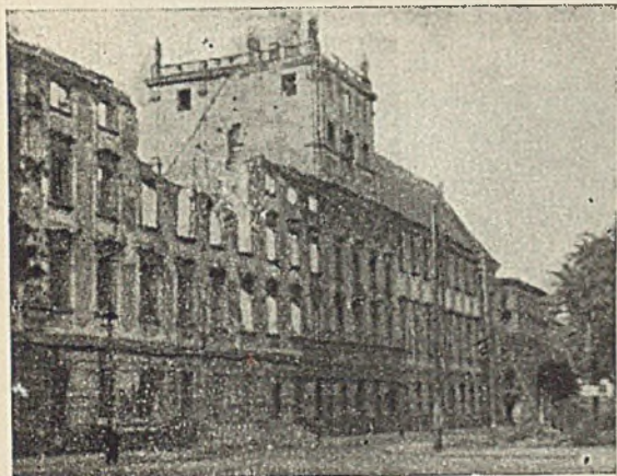
39. University main-building. War damage.
