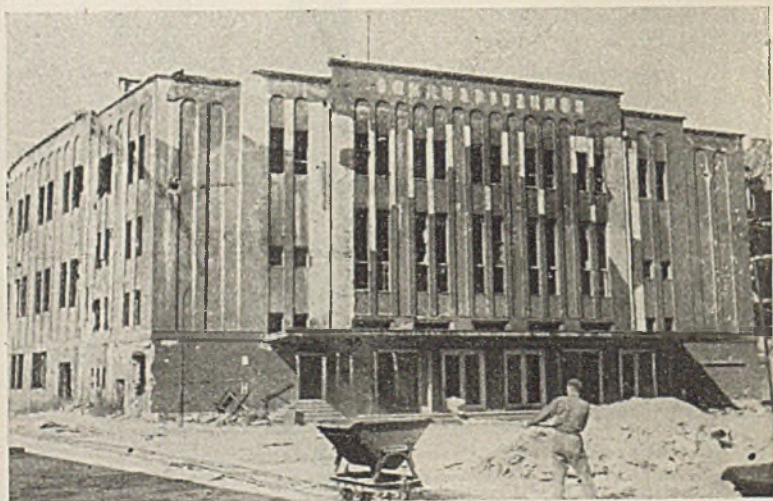
50. The fourth theatre of Wrocław was raised from ruins and dedicated to the play-wright Gabriela Zapolska.
