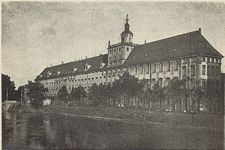
40. The same building after reconstruction.
