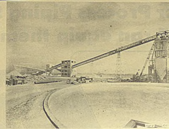
5 Dolomite from the quarry at Austin is transported by conveyor to the crusher house and then to storage bins
