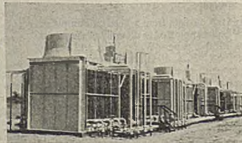
Radiator type coolers in a refinery
