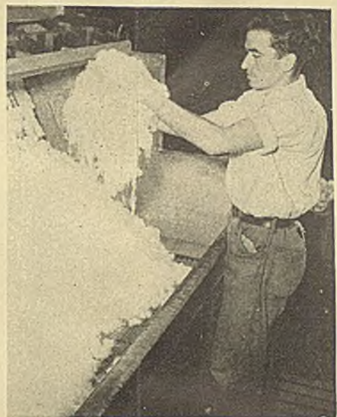
11 The short lengths are washed, desulphurized and bleached before drying
