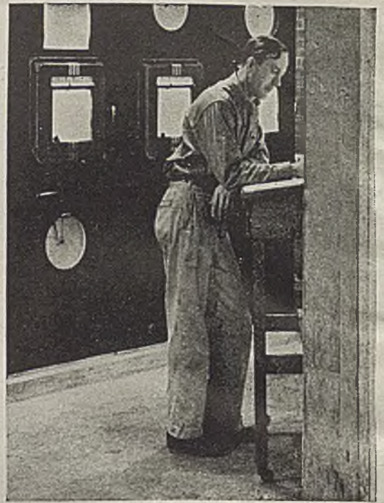
Left: Incoming operators at Butane Products Co., Port Neches, Texas, get a complete temperature history from the wide, easily-read strip-charts of Micromax Pyrometer Recorders. Above: Three of the 60 Micromax Recorders which provide accurate and reliable records of the important fractionating and dehydrogenating temperatures at this butadiene plant.
