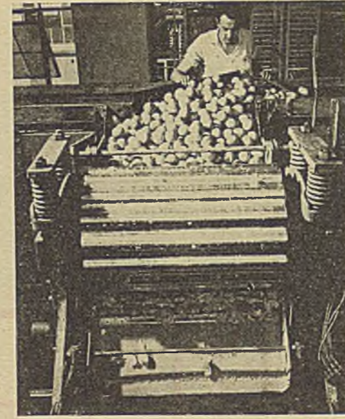
2 Fruit can be pressed between heavy corrugated rollers shown here
