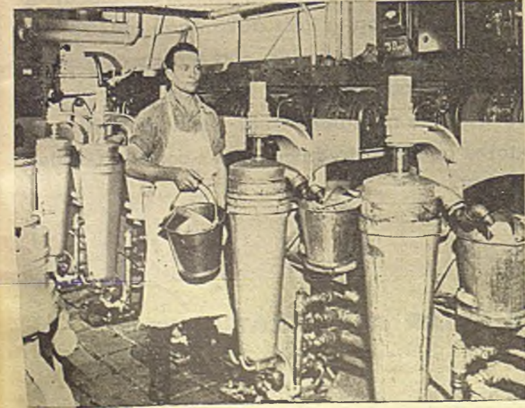
7 Separating orange oil (2 lb. from a ton of fruit) and juice
