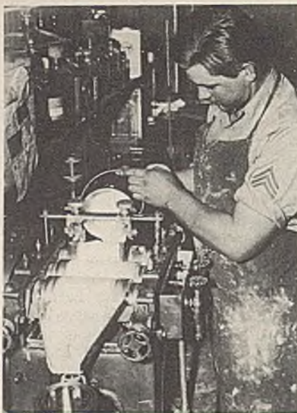
One of the new traffic paints using soybean oil goes through a three-roller paint mill
