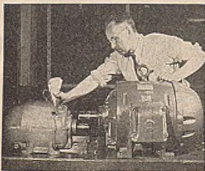
Both the smaller silicone-insulated motor and the conventionally insulated motor shown here developed 10 hp. at 1,750 r.p.m.
