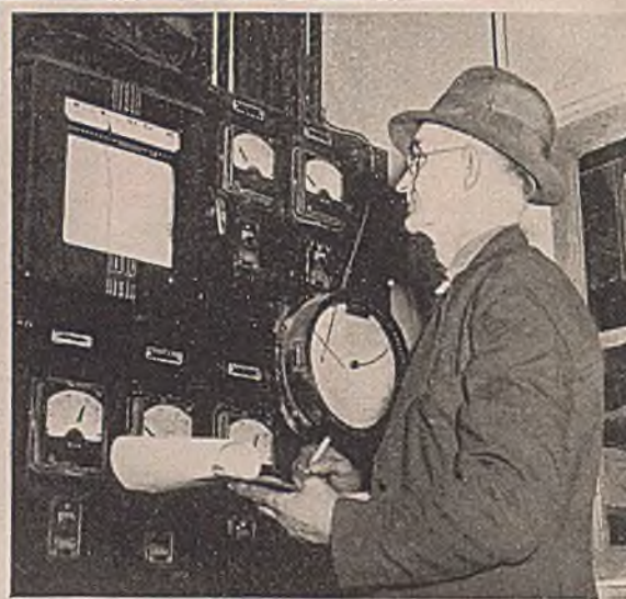
Above—Operator in Atlantic Refining Co.'s contact-process sulfuric acid plant, glances at Micromax Pyrometer Recorder to see trend of temperatures of \text{SO}_2 . Recorder in center is also for temperature; one at right shows strength of finished acid. Its range is 96.5 to 99.5% \text{H}_2\text{SO}_4 .
