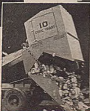
10 cu. yd. capacity waste or light materials handling body is shown at left.
