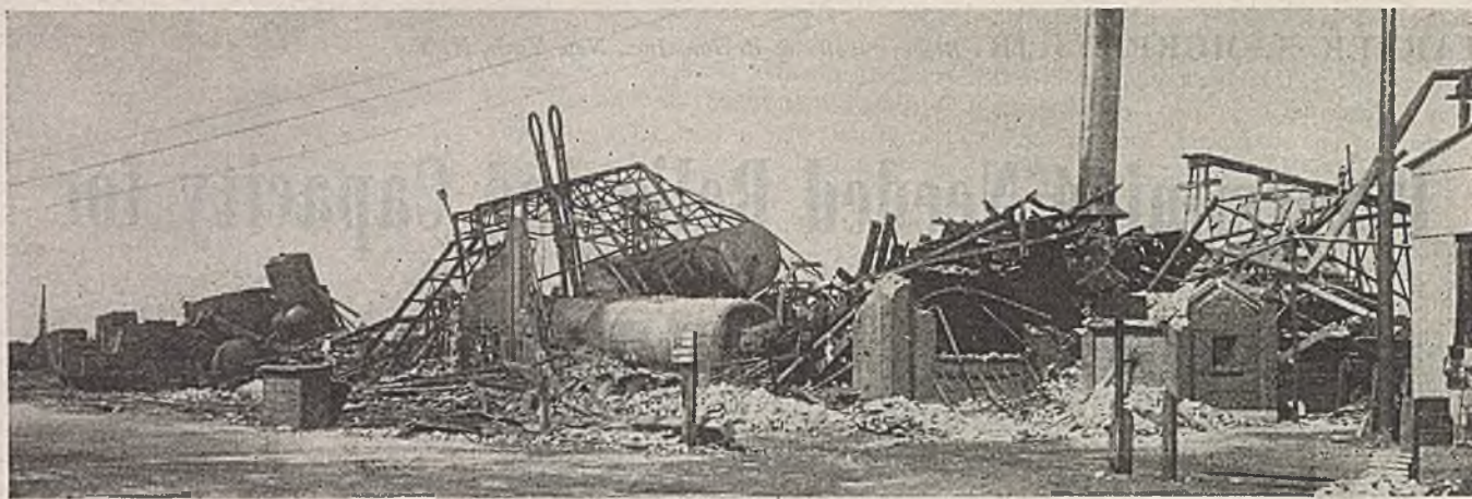
Fig. 1—Pressure rupture of a creosoting vessel after combustion of its contents caused this destruction
