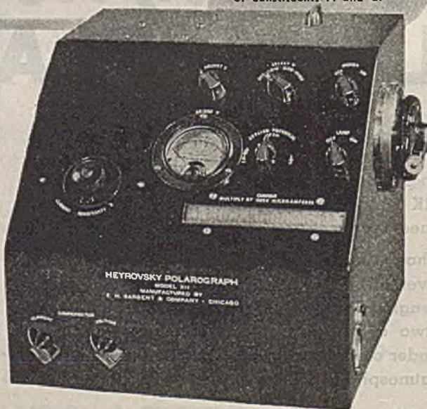
5-29301 POLAROGRAPH—Heyrovsky, American Model XII, Indicating-Recording, With Current Compensator. Complete with accessories. For operation from 115 volts, A.C. 60 cycle circuits .....$550.00
