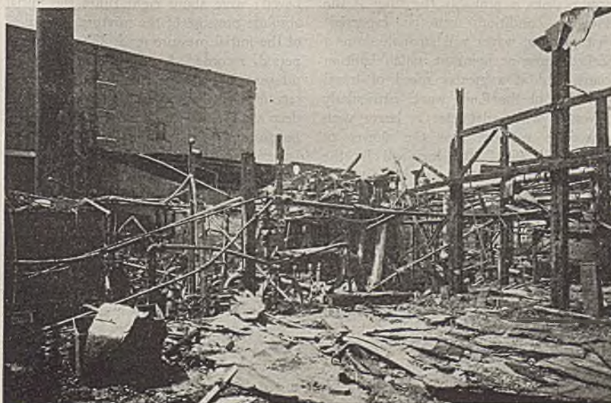
Fig. 2—Overpressure in a brine cooler released ammonia which became ignited, causing destruction of this plant by fire
