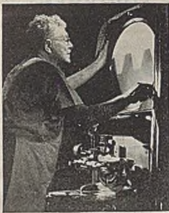
B&L Contour Projector magnifies tiny gear with accuracy to .0001"
