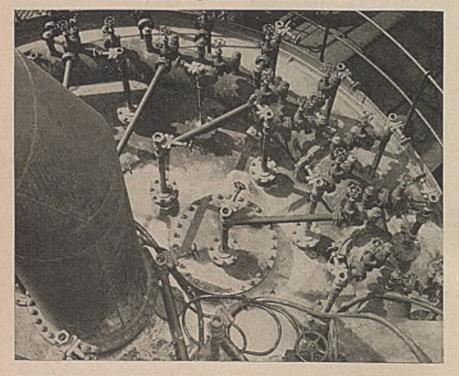
used in the autoclave and results in the melting of the sulphur which separates to the bottom half of the autoclave, leaving the scum and impurities on the top. Having been thus separated from the water and other impurities, the sulphur may be drained into a cast iron mold and allowed to solidify, or processed by a newer method developed at the Ford plant. In either case, the impurities are blown off to a steel tank to be reworked.
