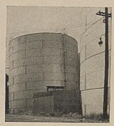
After 11 years, the tanks had settled 5 ft. on one side and 2<sup>1</sup>/<sub>2</sub> ft. on the other, but the foundation remained in a straight plane
