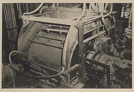
Fig. 1--No. 1 Syncro-Drum filter in U. S. Vanadium Corp. plant
