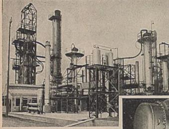
Cracking still tubes of 18-8 chromium-nickel stainless steel withstand high temperatures and pressures.
