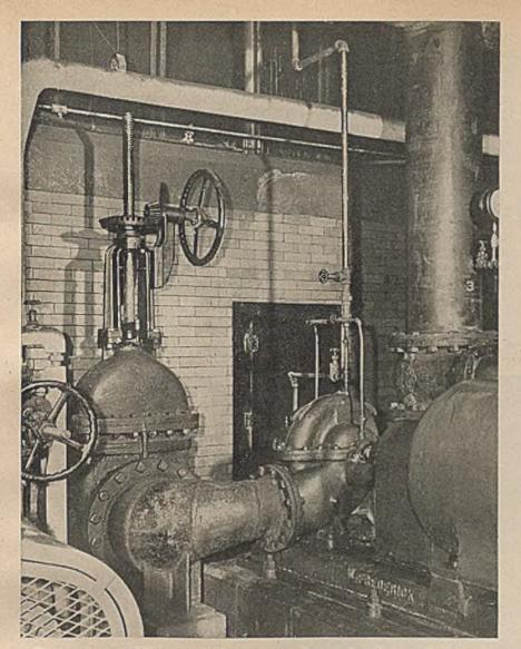
There are two 125-hp. centrifugal pumps in continual operation transferring the foul Thylox solution from the absorbers to the reactivation equipment
