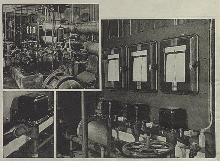
Typical views in the filter plant, Finishing Division of Arkwright Corp., Fall River, Mass. The three Micromax Recorders show, left to right, the pH of finished water at the clear well; pH of raw water coming into filter plant; pH of water just after alum and filters. Note electrode unit at left.
