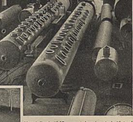
Vessels lined with 12 per cent chromium steel withstand corrosion, and save weight.
