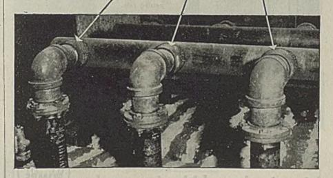
• On this piping installation the three branch pipe outlets were installed quickly and easily by the WeldOlet method. The elimination of any templates or the need for any cutting, forming or fitting, speeded and simplified the installation.
