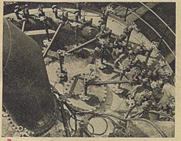
2. Thylox solution is fed to the absorber sprays through a ring manifold. Absorbers are 90 ft. high
