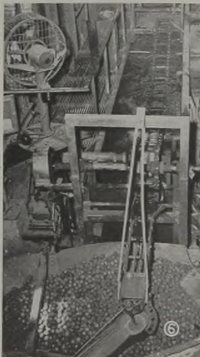
Fig. 6—Grinding balls being conveyed through quenching medium
