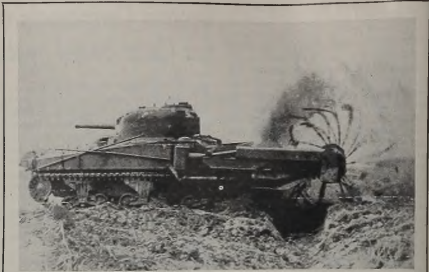
MINE FLAIL: The "Scorpion," Britain's flail tank, sees action in Normandy. The tank is equipped with chains which extend from a boom and revolve rapidly beating the ground in front of the tank and detonating buried mines. NEA photo
