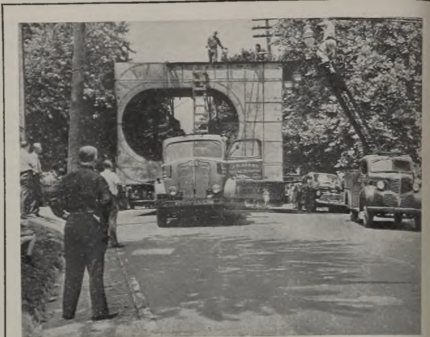
HIGHWAY CONFUSION: This huge 20-ton steel stack is shown on the last stage of its six day journey to the Philadelphia navy yard. Traffic was halted on the highways while electricians took down and replaced telephone and electric wires on the road. Because of such interference the stack required six days to go only 60 miles. NEA photo
