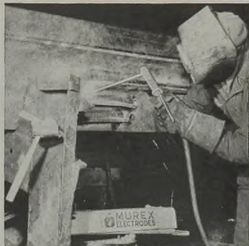
THE DRAFT SILL ASSEMBLY of a freight car is being welded with Murex Electrodes in the plant of Pullman-Standard Car Manufacturing Company. Downhand rods are used because they are ideal for long, horizontal fillets and deposit sound X-ray clean weld metal at a rapid rate.
