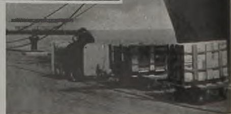
(Right)—Delivering palletized loads at shipside. One man with fork truck unloads car (illustrated above) faster than 8 to 10-man gang
