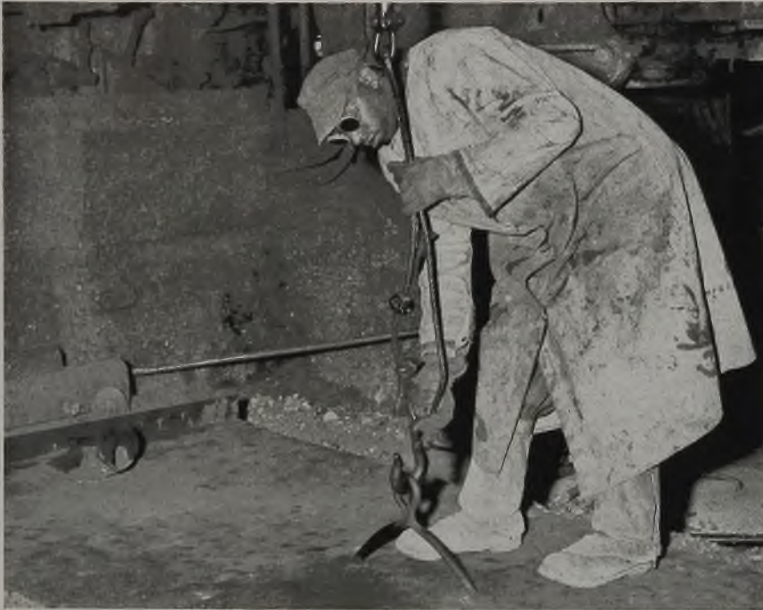
Fig. 1—(Above)—Method used in placing platform in position and removing after tap hole has been drilled
