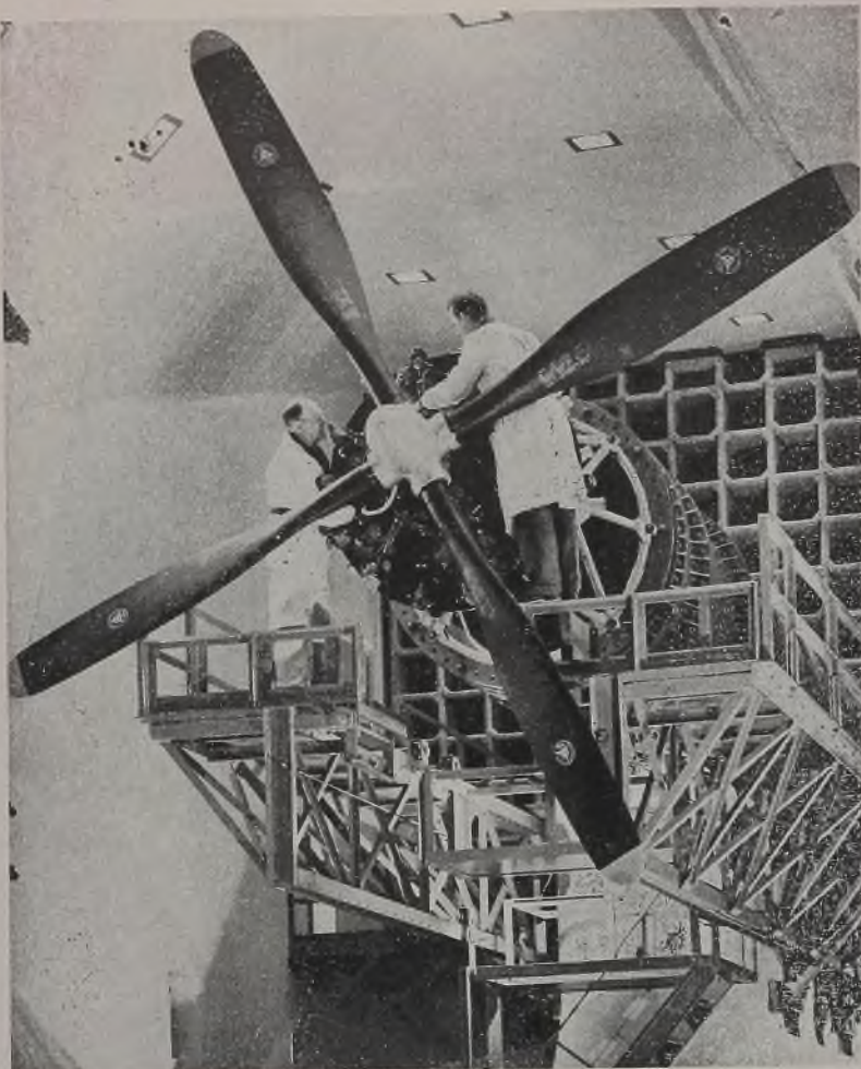
ABSORBS 3000 HORSEPOWER: Claimed to be the largest 4-blade hollow steel propeller in quantity production in this country, this 16-foot, 8-inch propeller being produced by Curtiss-Wright Corp., is designed to absorb 3000 horsepower. Above it is shown in a test cell at the company's Caldwell, N. J., plant
