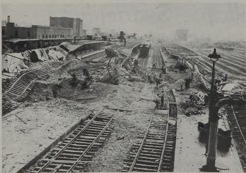
Uprooted tracks, blasted rolling stock and destroyed engine sheds mark the rail center at Caen, France, as Allied engineers move in to repair their own destruction. Rehabilitation of devastated areas will require a huge quantity of steel. NEA photo
