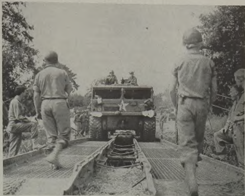
AMERICAN INGENUITY: On the heels of rapidly advancing American forces in France, Yank engineers are quickly repairing and rebuilding roads and bridges wrecked by the retreating enemy. This prime mover pulls artillery equipment over a treadway bridge speedily erected by Americans. NEA photo
