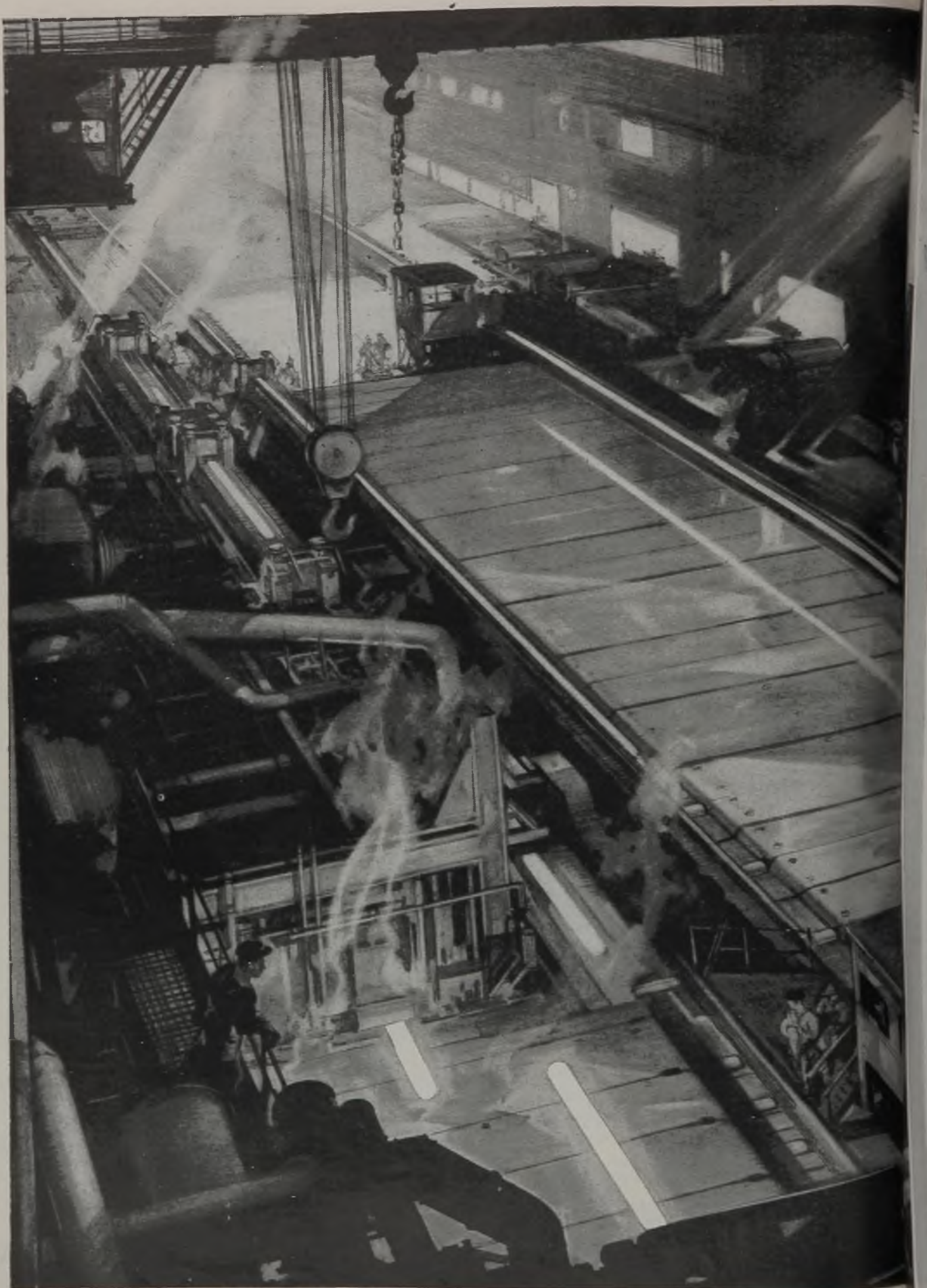
FROM AN ORIGINAL DRAWING AND SKETCHES BY ORISON MACPHERSON, AT JAL PITTSBURGH WORKS
