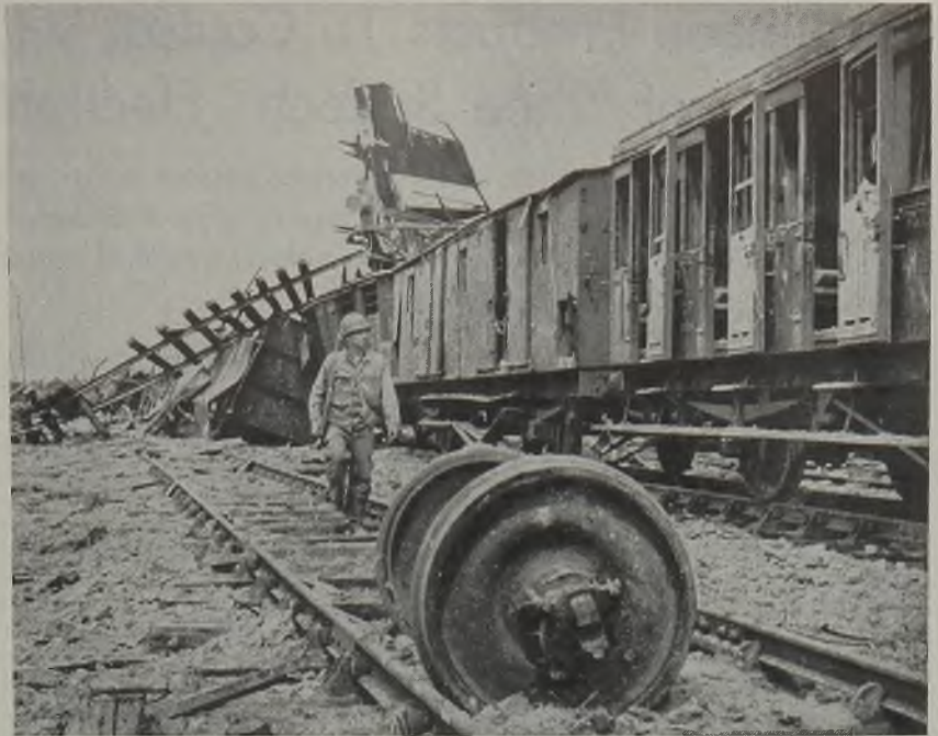
Much American-built equipment will be required to replace European railway rolling stock destroyed by Allied bombing or by Nazi demolition. Above is shown wreckage caused by American bombings near Carentan, France, during the invasion. NEA photo
