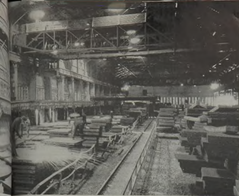
(Above)—Three-kilowatt mercury tubes provide adequate light on plate scarfing floor, Geneva Steel Co., Geneva, Utah. (Westinghouse photo)
