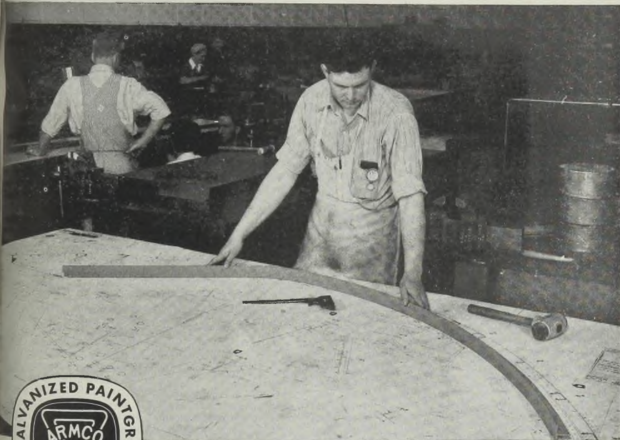
Checking contour of a body frame section.
