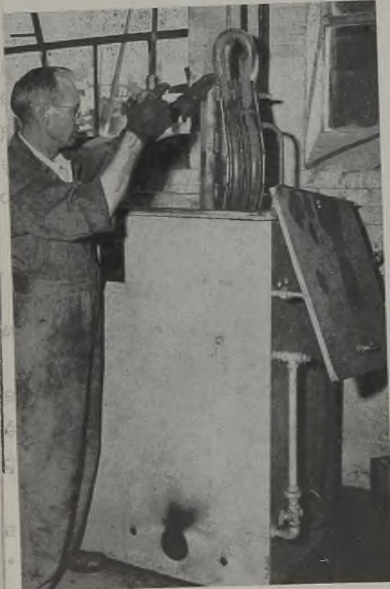
(Left)—Chemical degreasing tank where all accessory parts are cleaned before painting
