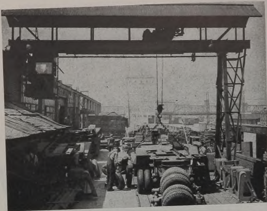
(Above)—Final assembly is done outdoors under single-legged gantry as shown here. Front dolly, rear bogies, loading ramps, tools, and lashing gear come together at this point
