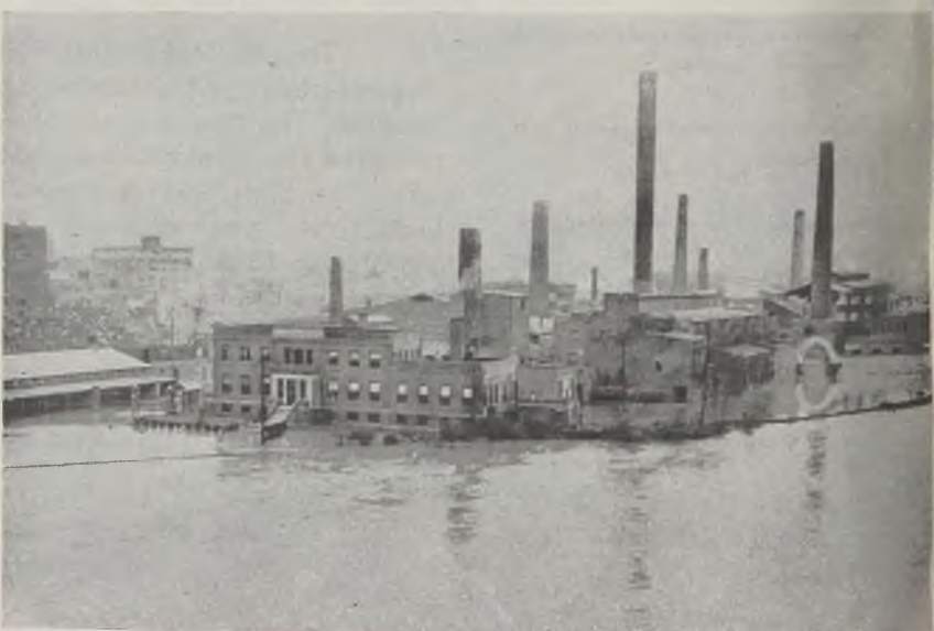
No smoke pours from the stacks of this smelter at Omaha, Nebr., as the Missouri river leaves its banks in the 1943 flood. Millions of dollars of property damage have been caused by the annual rampages of the Missouri, contra which now has been proposed to Congress. NEA photo
