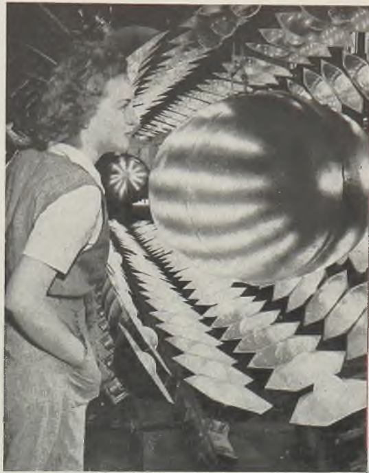
Fig. 4—Infra-red heat lamps baking exterior and setting interior finishes
