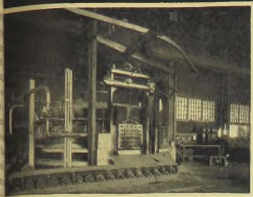
This type of Salem furnace not only gives you very close control of the heating rate, but also of the atmosphere. Pictured above is a furnace used to heat treat high carbon and alloy steels.
