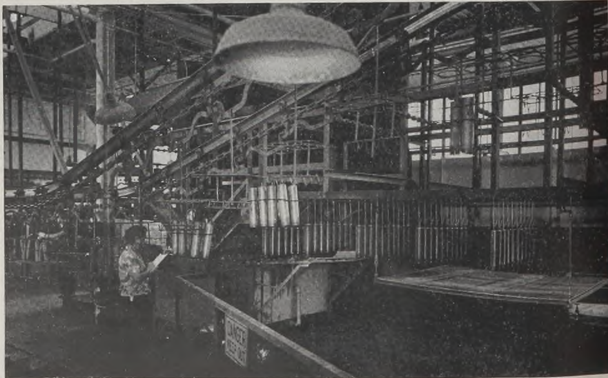
Here bank of 10 cartridge cases is passing over first set of detearing screens. Cases are grounded to conveyor, forming one electrode; expanded metal screen forms other electrode. Potential of 85,000 volts between the two forms powerful electrostatic field which rapidly dissipates tears or clinging beads of varnish on drain-off points of the work. Data and photos from Pittsburgh Plate Glass Co., Pittsburgh
