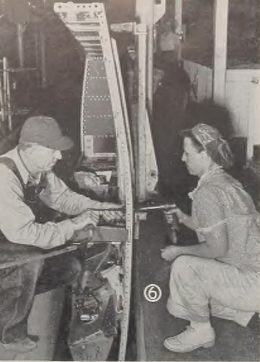
Fig. 6—Workers at North American Aviation's Inglewood plant rivet and buck Hi-Shear rivets with two rivet guns instead of single gun and bucking bar
