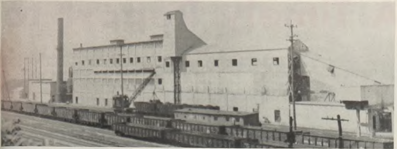
General view of Wheeling Steel Corp.'s sintering plant at Steubenville, O. Raw material bins are housed at right of skip hoist; sintering department at left
