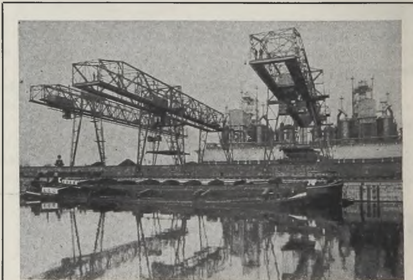
KRUPP BEFORE BOMBINGS: Just before American and British bombers started dropping heavy loads of explosives on the Krupp armament works at Essen, Germany, this photo shows the docks and blast furnaces at the leading Nazi munitions plant. NEA photo
