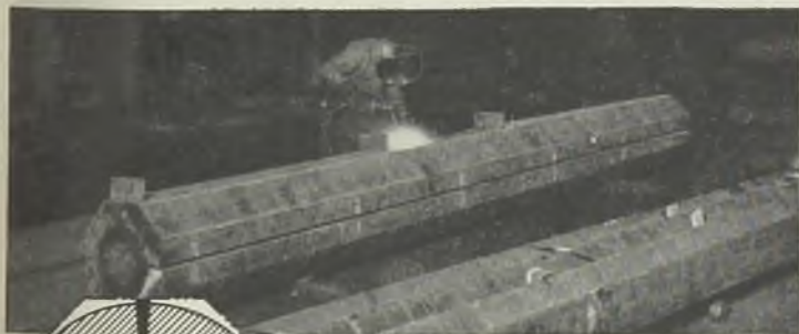
This huge column, one of four for a 3300-ton hydraulic press, was fabricated from four segments by arc welding because of the inability of steel foundries to produce a cast column with a 14" bored hole straight enough to allow a 13" rod to pass through it. Murex downhand electrodes were used, starting with 5/32" rods and changing to 5/16" size as the width of the joint increased.
