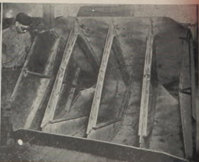
Fig. 4 (Below)—Interior construction detail of end section showing method of welding reinforcement members
