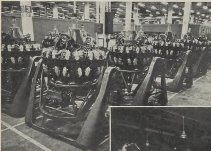
Production of the new Wright Cyclone 18 engines of 2200 horsepower, above, for super bombers and other long-range planes will be increased 750 per cent in 1944
