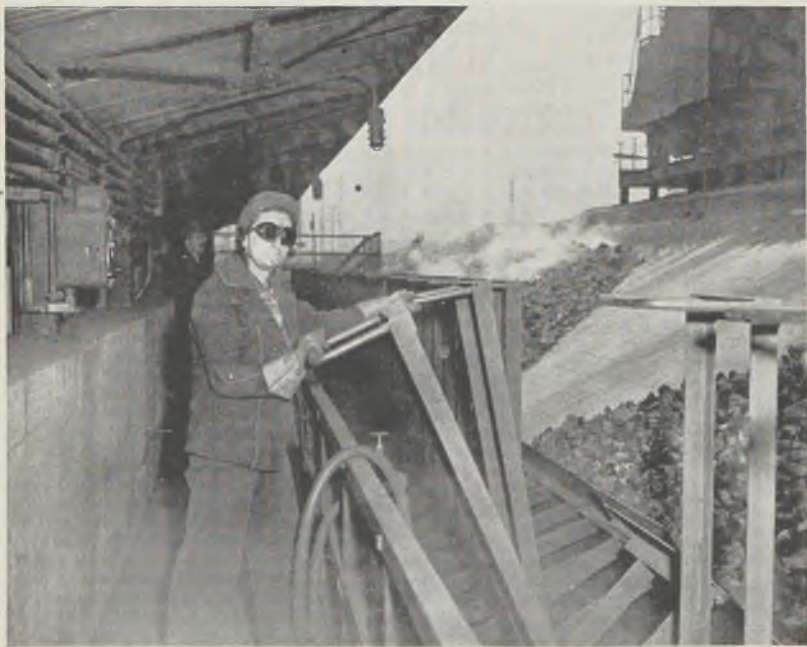
NEW COKE PLANT: Spurred by heavy demand for steel and chemicals for war, the new coke plant of the Pittsburgh Steel Co. at Monessen, Pa., is operating at capacity. Above, a woman worker operates device to drench and cool the hot coke with water
