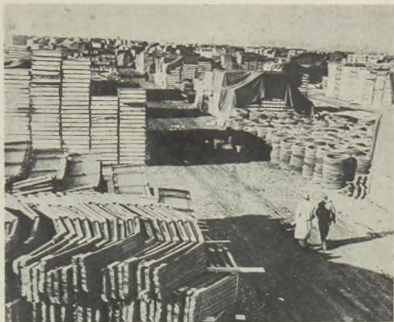
INVASION BOUND: Earmarked for Europe are these stacks of prefabricated barracks and steel material for hut construction at a United States engineering depot in England. Acme photo
