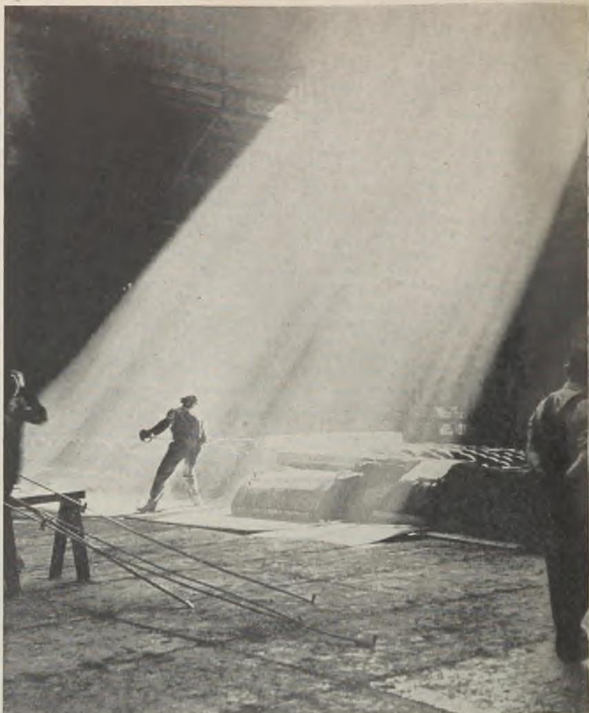
More than one-third of the nation's ship plates produced in 1943 came from the mills of the United States Steel Corp. This photo from the corporation's annual report shows a workman turning a slab broadside preparatory to further rolling on a 140-inch sheared plate mill
