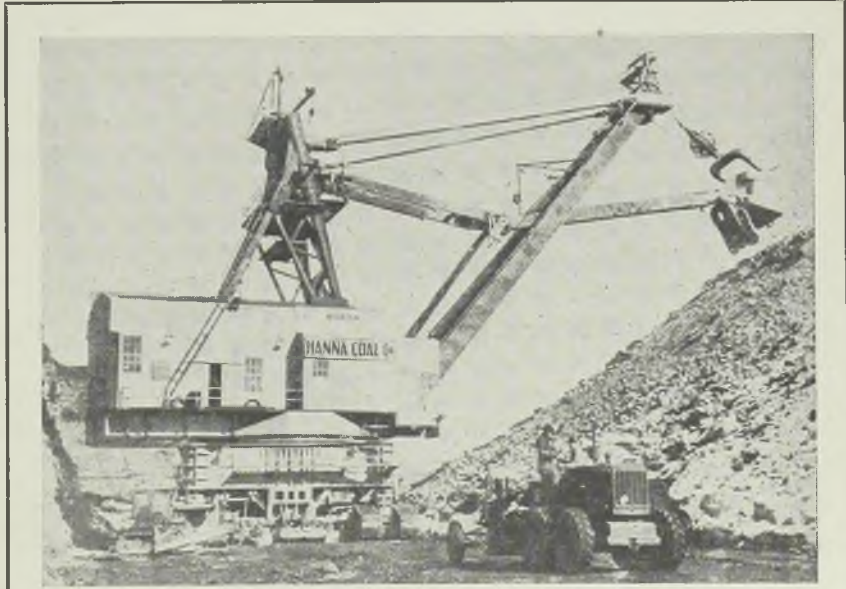
BIG SCOOP: One of the largest shovels in the world, built at Marion, O., is shown in operation at the Hanna Coal Co.'s strip mine at Georgetown, O. It weighs 16,000 tons. The dipper has 35 cubic yards capacity, and will carry 20 per cent more. Tractor treads are 6 feet high, and the whole structure is more than three stories in height. NEA photo
