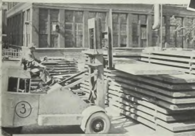
Fig. 4—Battery-powered pallet truck with platform on forks safely handles heavy spools of wire over upper floors too light for heavier trucks
