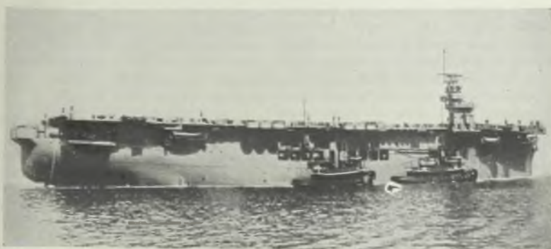
CONVERTED: The tanker NEW ORLEANS has been converted into an escort aircraft carrier by a Bethlehem Steel Co. shipyard. The conversion job involved removal of the tanker's superstructure and the bulkheads in the tank spaces and installation of carrier equipment, including two platform elevators
