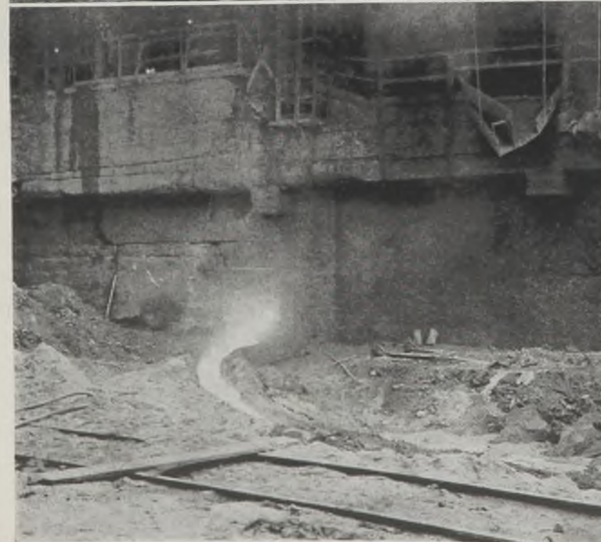
Fig. 1—Using an oxygen lance in tapping a salamander during a blowout of a Valley stack
