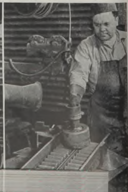
Fig. 11—Right: Gravity roller conveyors carry work from station to station. Note flexible hose of system used to exhaust welding fumes
