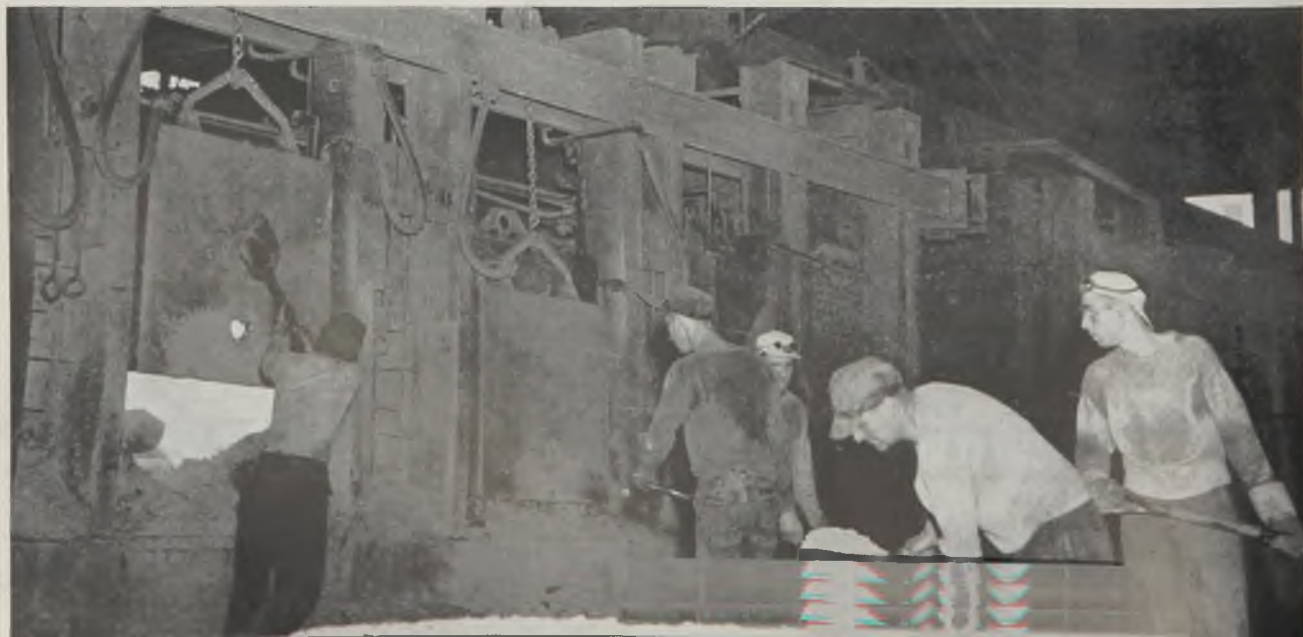
Below, water-cooled charging doors on open-hearth furnace
