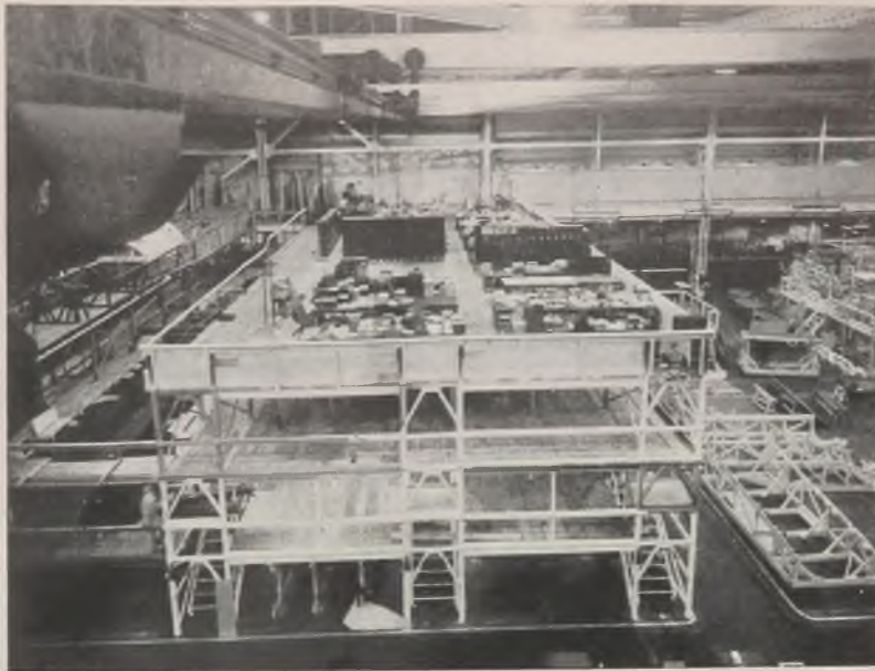
SPACE CONSERVER: One of the two emergency office buildings at the Glenn L. Martin Co., Baltimore, which have been converted from PBM hull fixtures that no longer were needed as result of improved assembly methods. Created as an emergency measure to meet a critical floor space shortage, the new offices will house electrical workers and light manufacturing groups
