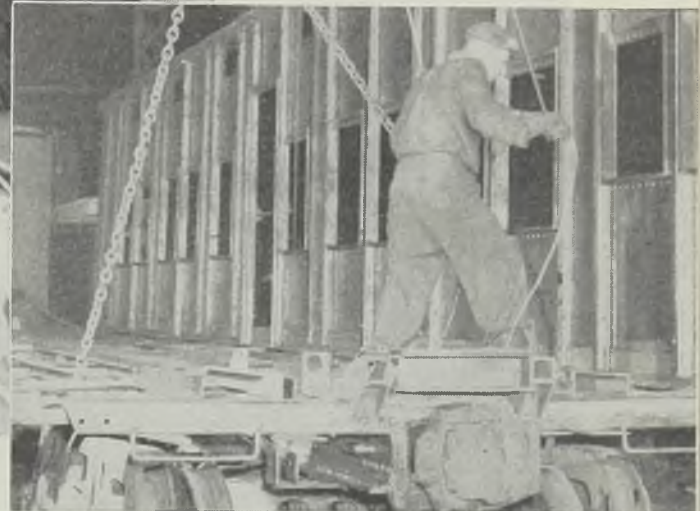
Sub-assemblies speed up the job of building 1,200 new troop sleepers.
