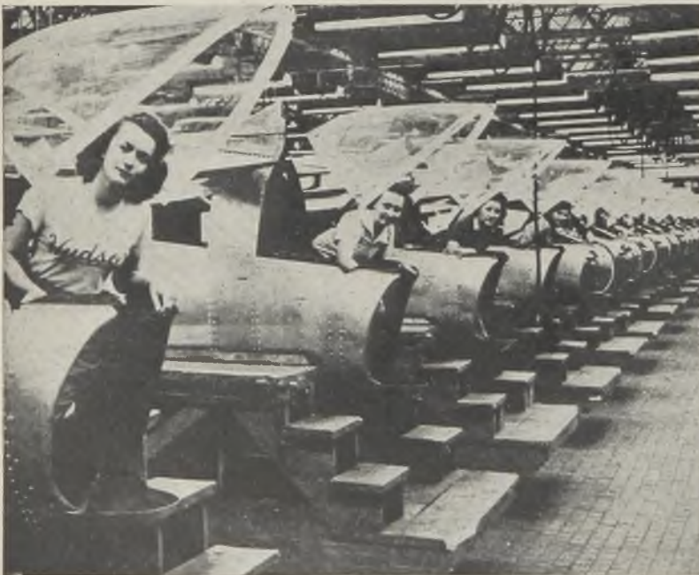
PACK LETHAL BLOW: Four girls standing beneath the plastic bonnets in the fuselage sections of the Martin B-26 Marauder bombers built in a Hudson plant in Detroit give some idea of the size of the mechanism that loads and fires the hard-hitting tail guns. The secret mechanism will be installed after final inspection of the space the girl workers occupy
